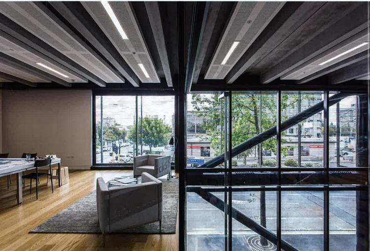
Sustainable design solutions are seen on the building's interior, too. Precast double-tee concrete at ground floor with open-plan workspaces, the ceilings are exposed to increase thermal mass while further visually expressing the structural make-up of the building.
